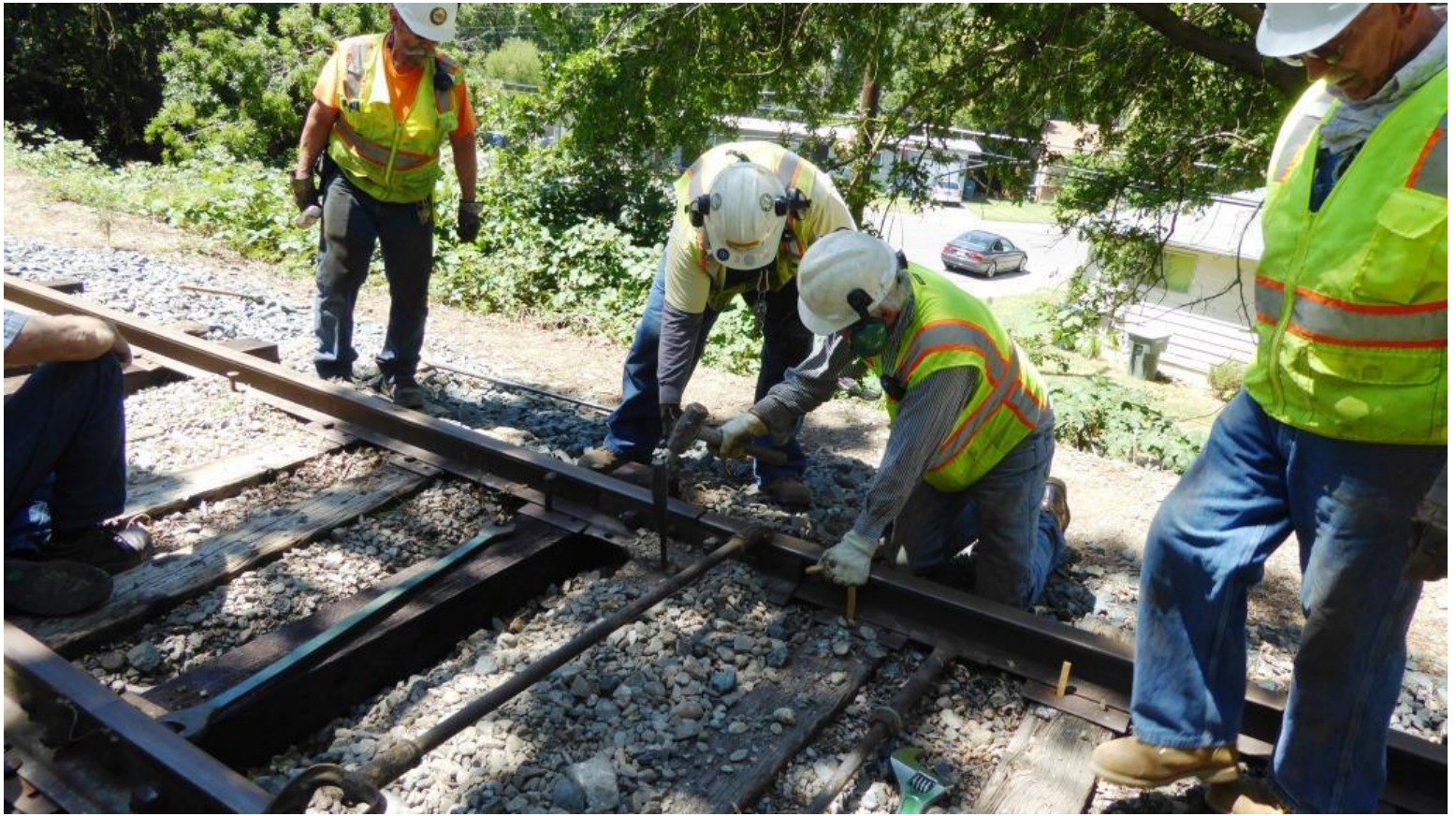
Mike F. and Steve plug spike holes in the ties where spikes were pulled to allow the necessary movement of the west rail back into gauge
