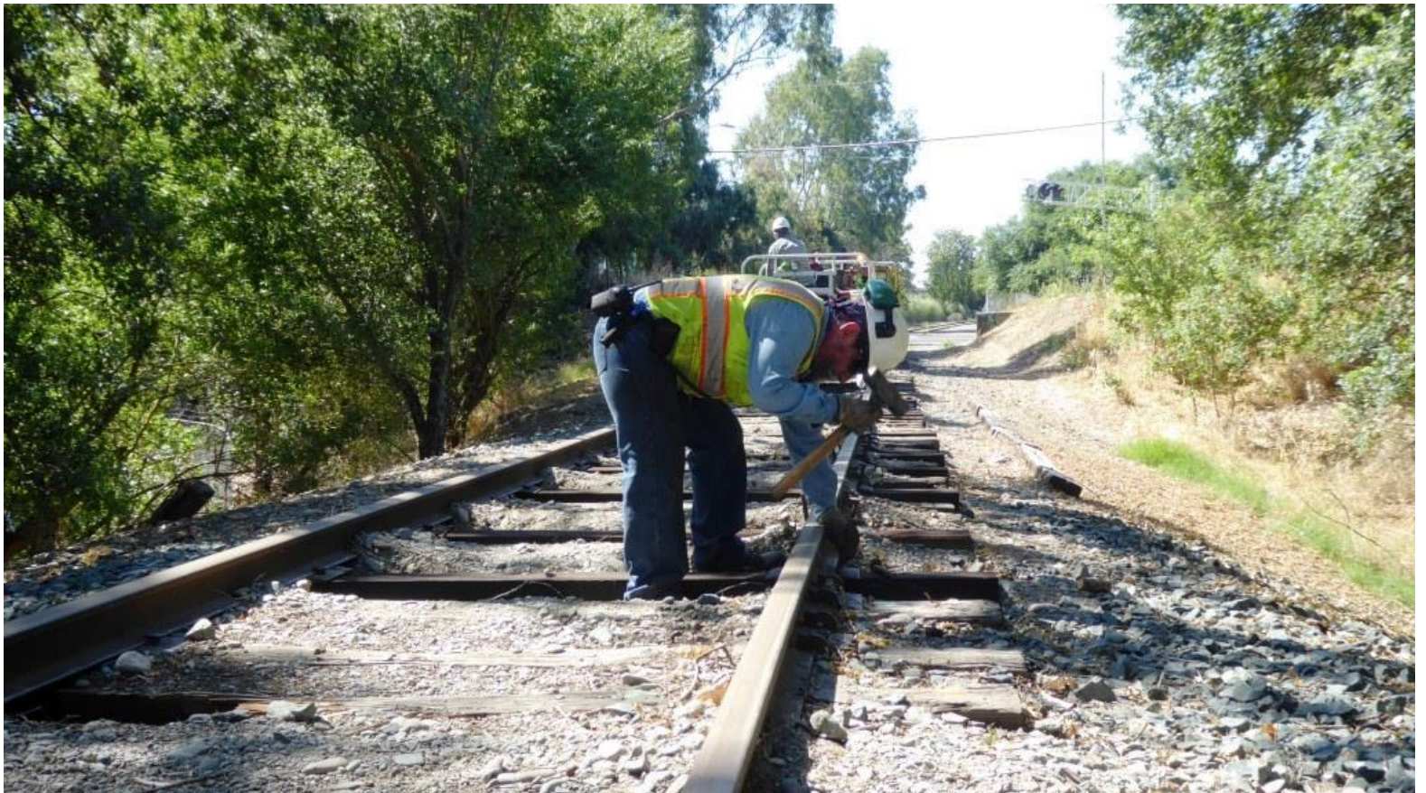
Joe sets spikes in areas where the gauge is good
