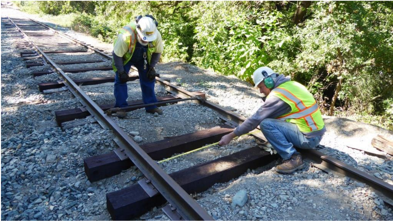
Clearly, the pipe-gauge will not seat on the rail because the gauge is narrow so, Steve takes a measurement with a tape
