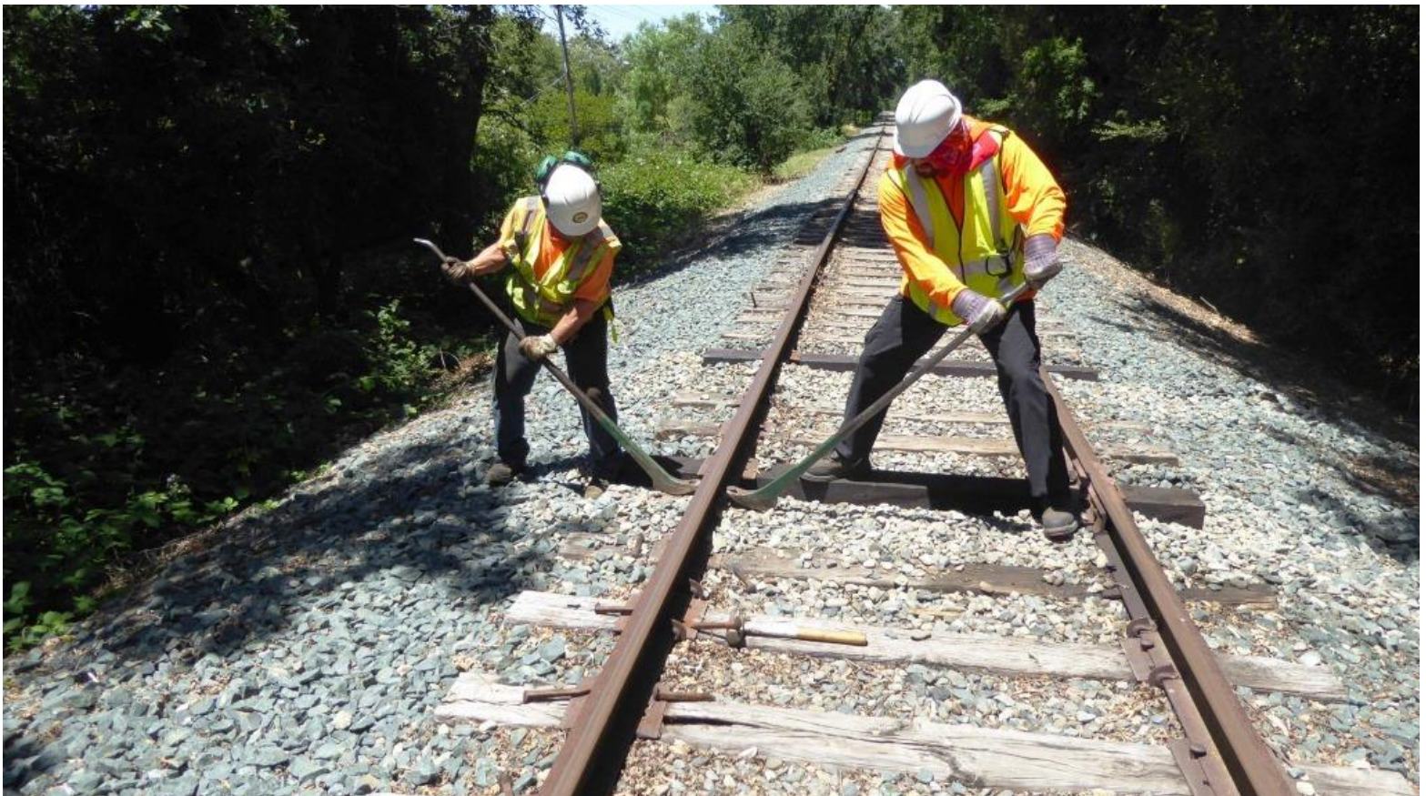
...As Joe and Jose pull spikes in the old ties to allow the west rail to move when gauged
