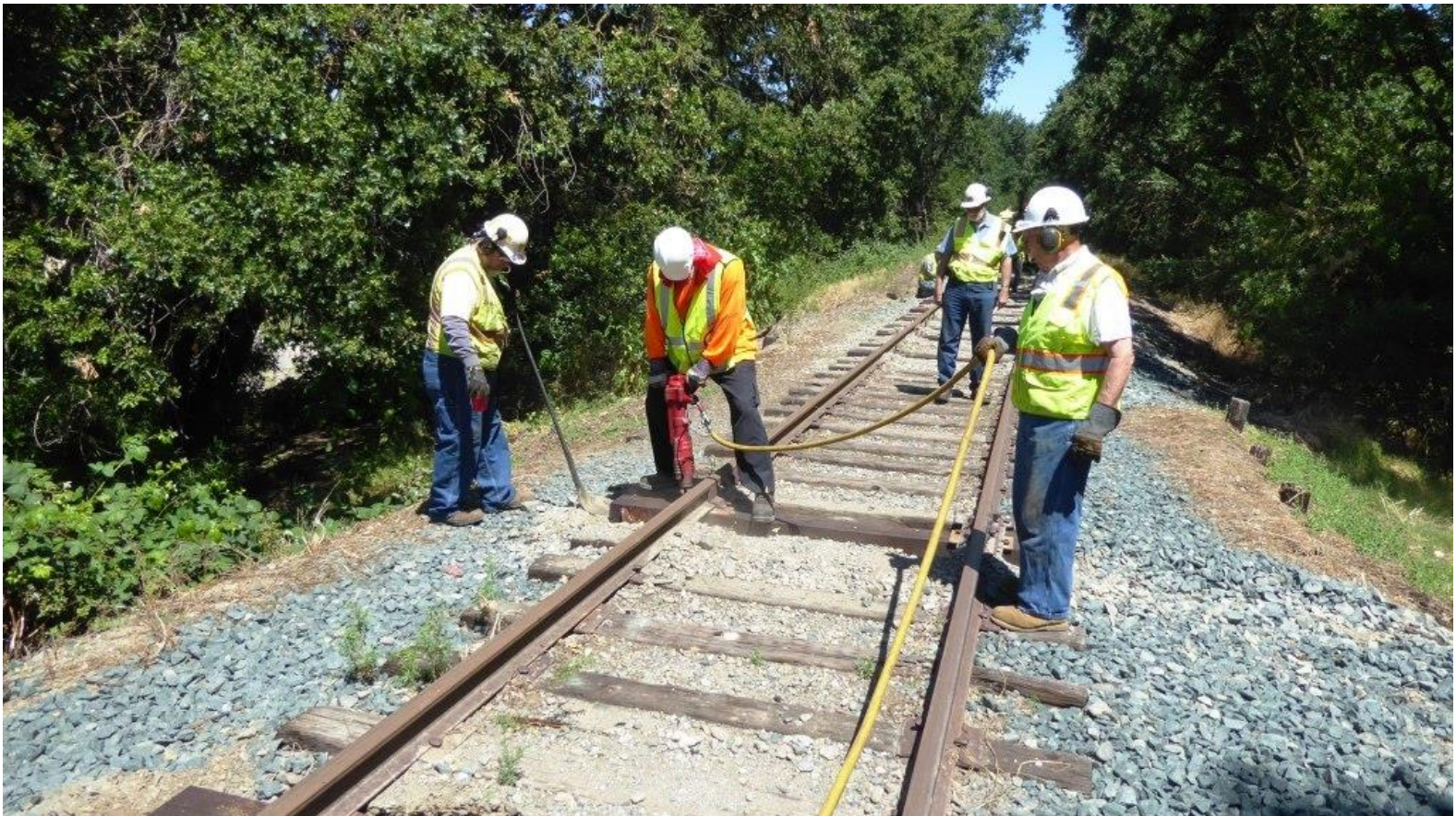
Mike F. nips the rail as Jose drives the spike while Clem handles air-hose duty
