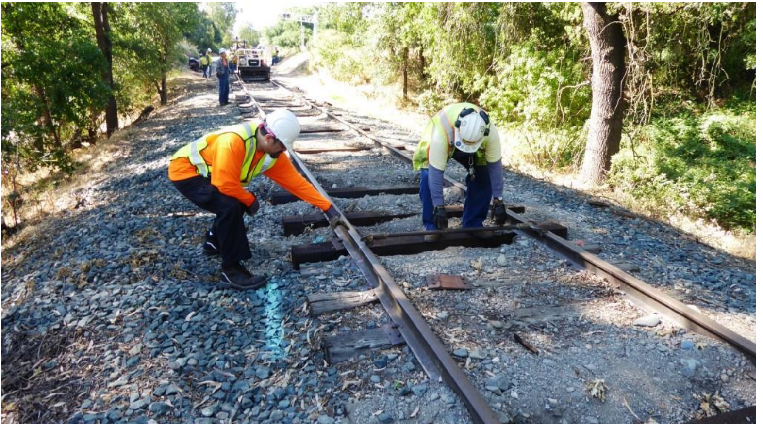
Down on the Sutterville Line, Jose and Mike F., using the pipe-gauge (measurer), identify a narrow spot
