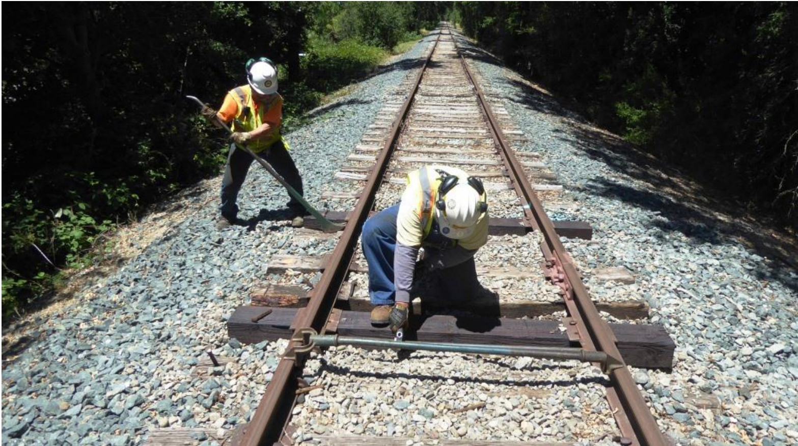
Joe pulls spikes ahead of Mike F. and the manual gauger
