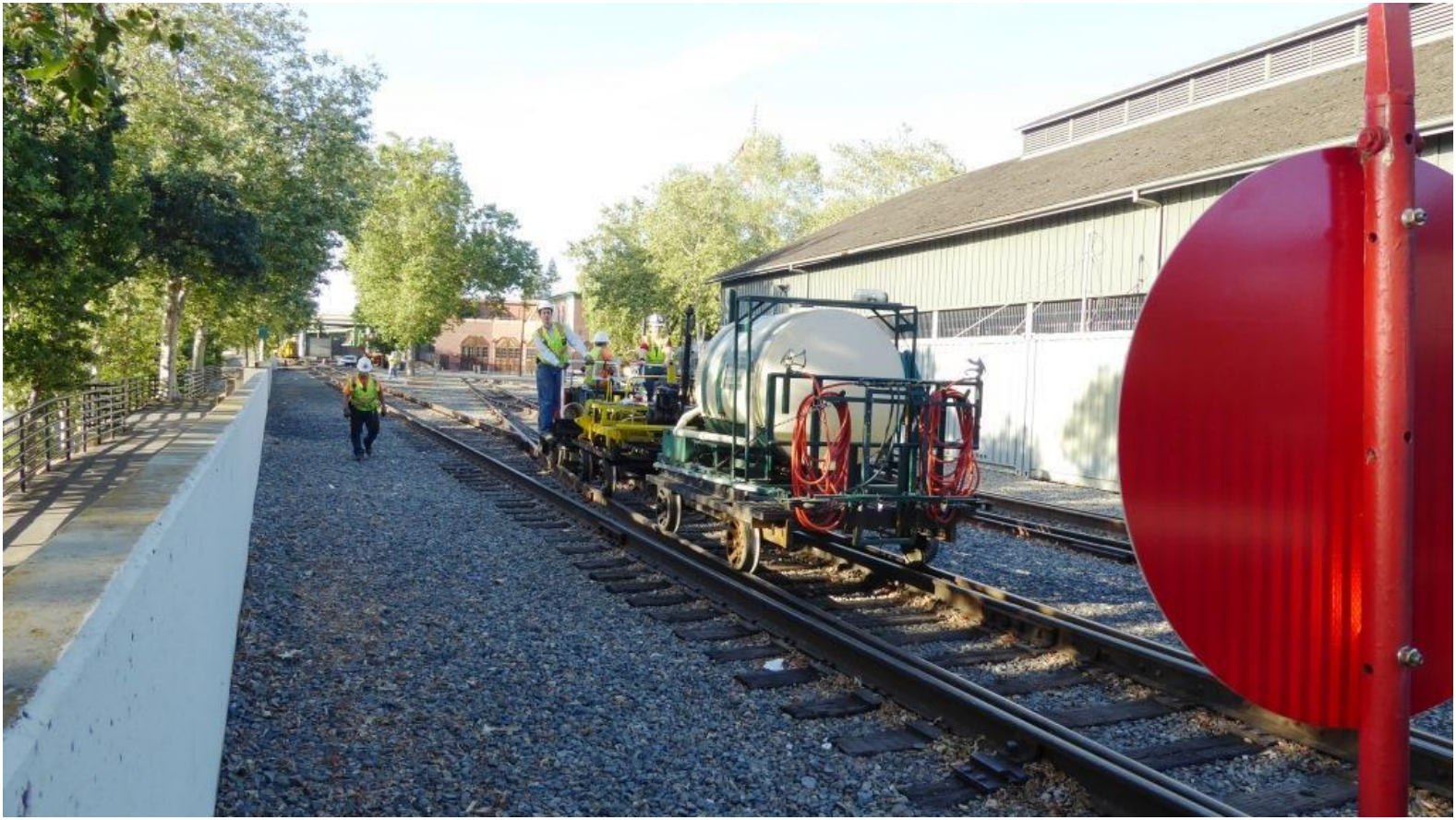
Weston "calls the shove" as the spray-rig and rail-lifter carriage are moved onto the Old Main
