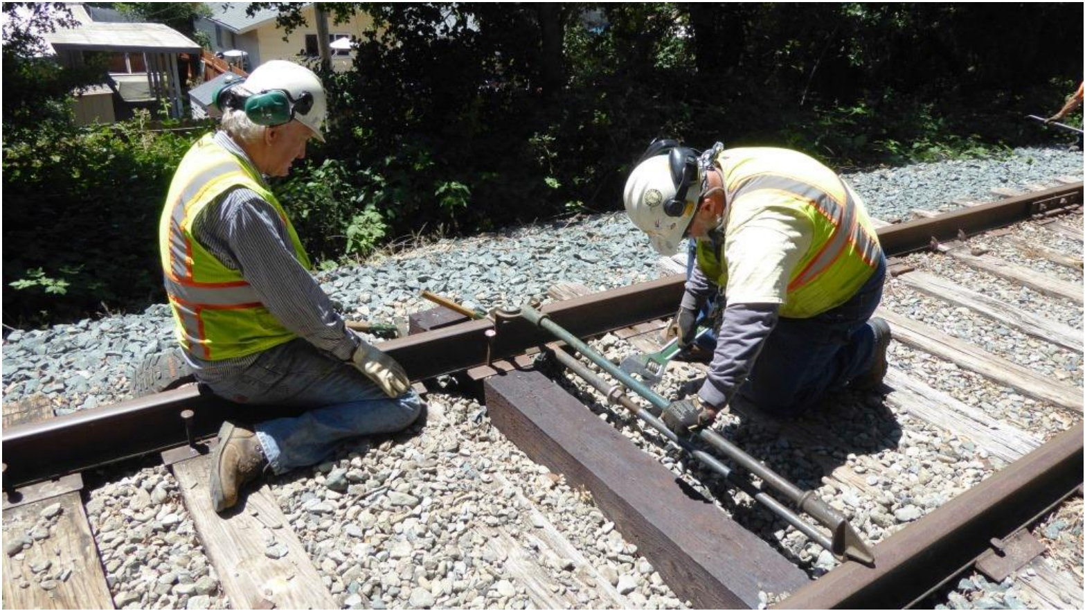
Steve and Mike continue with re-gauging the track...
