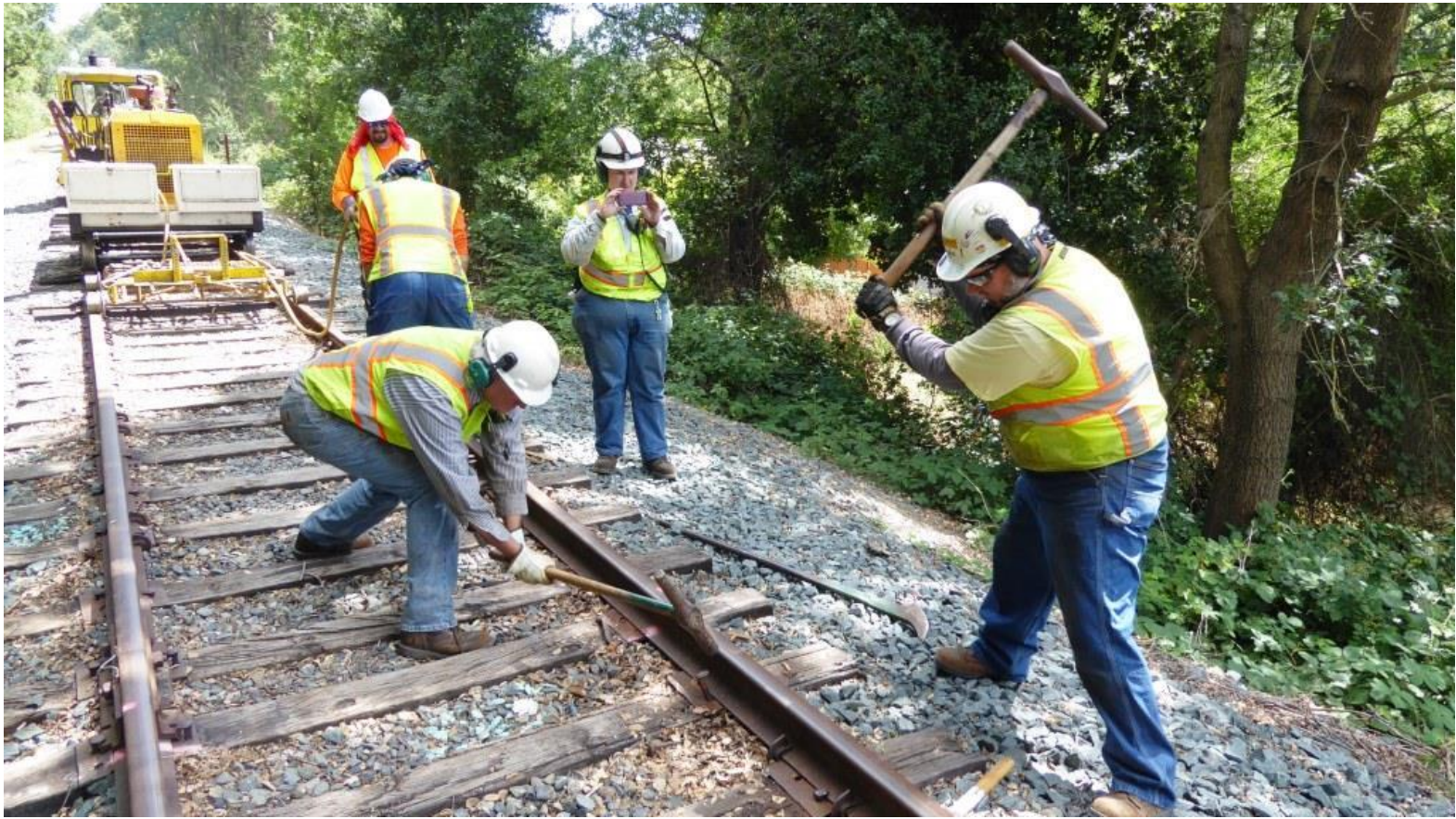
Steve and Mike F. are driving the same spike, hitting it in alternating swings of their spike-mauls
