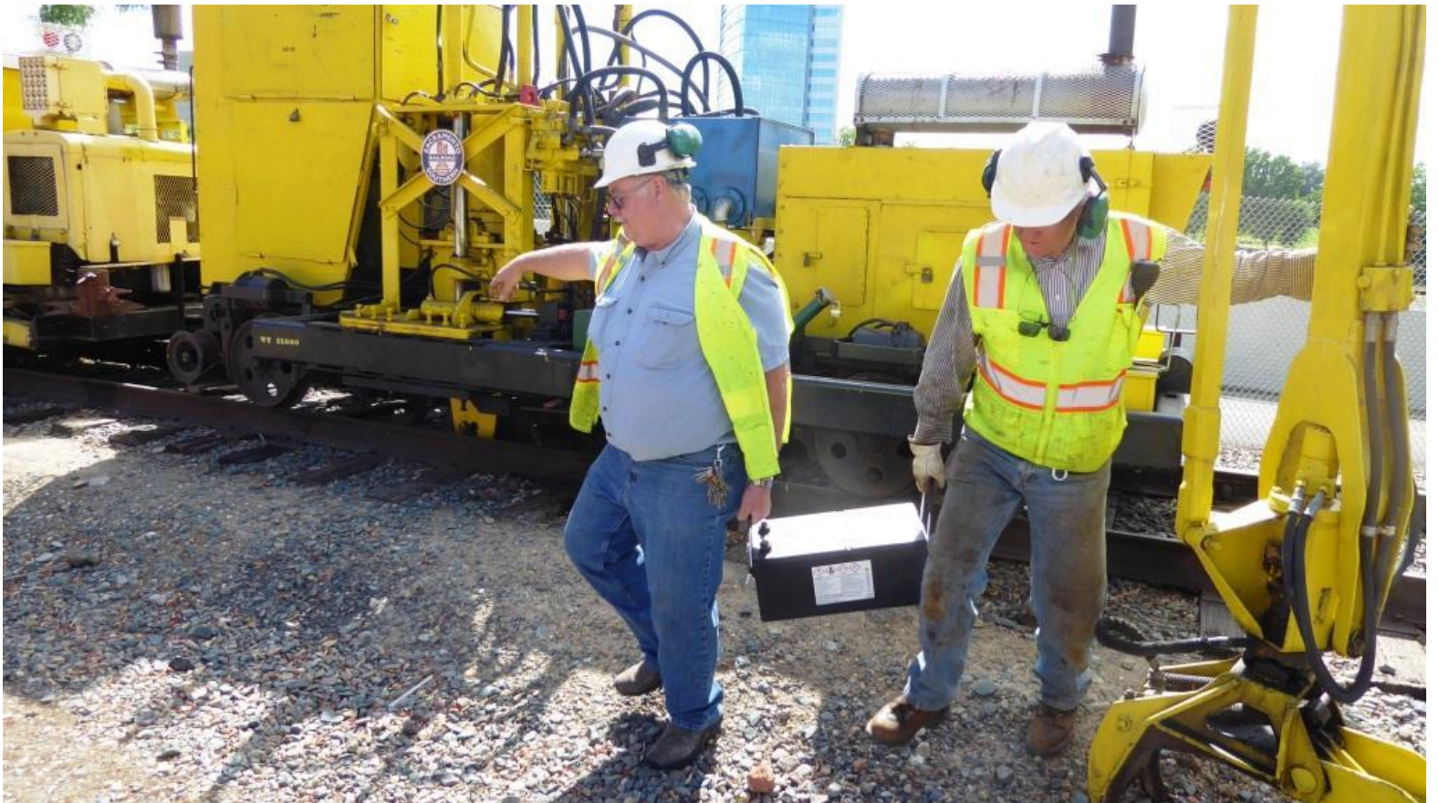
At the end of the day, Chris C. and Steve removed the battery from the tie-shear for charging
