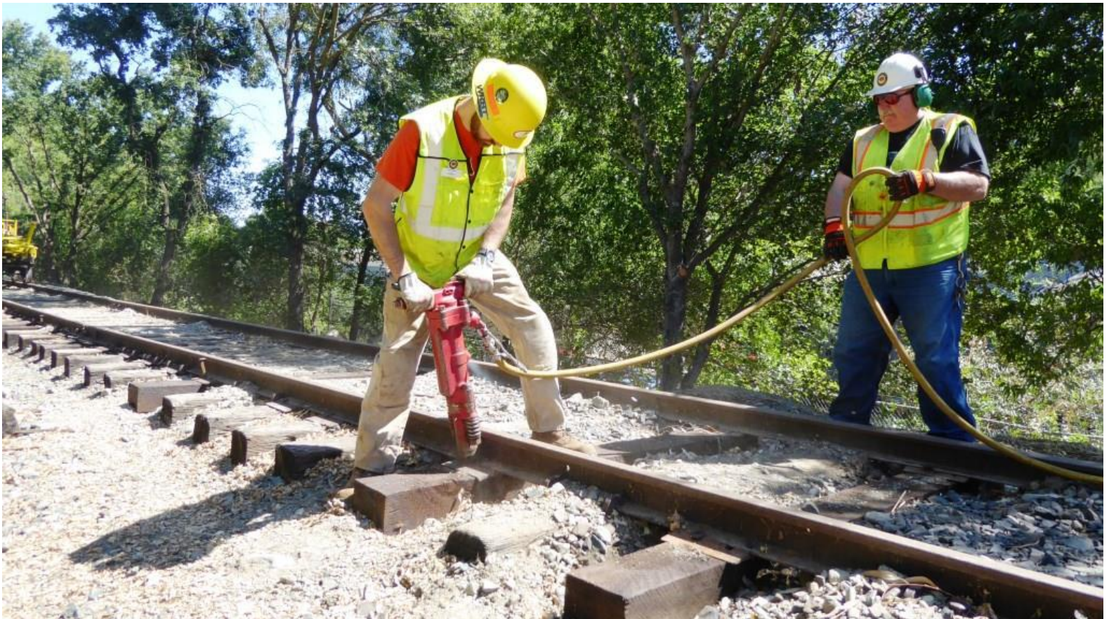
Chris M. takes the on the pneumatic spike-driver as Harry guides the air-hose
