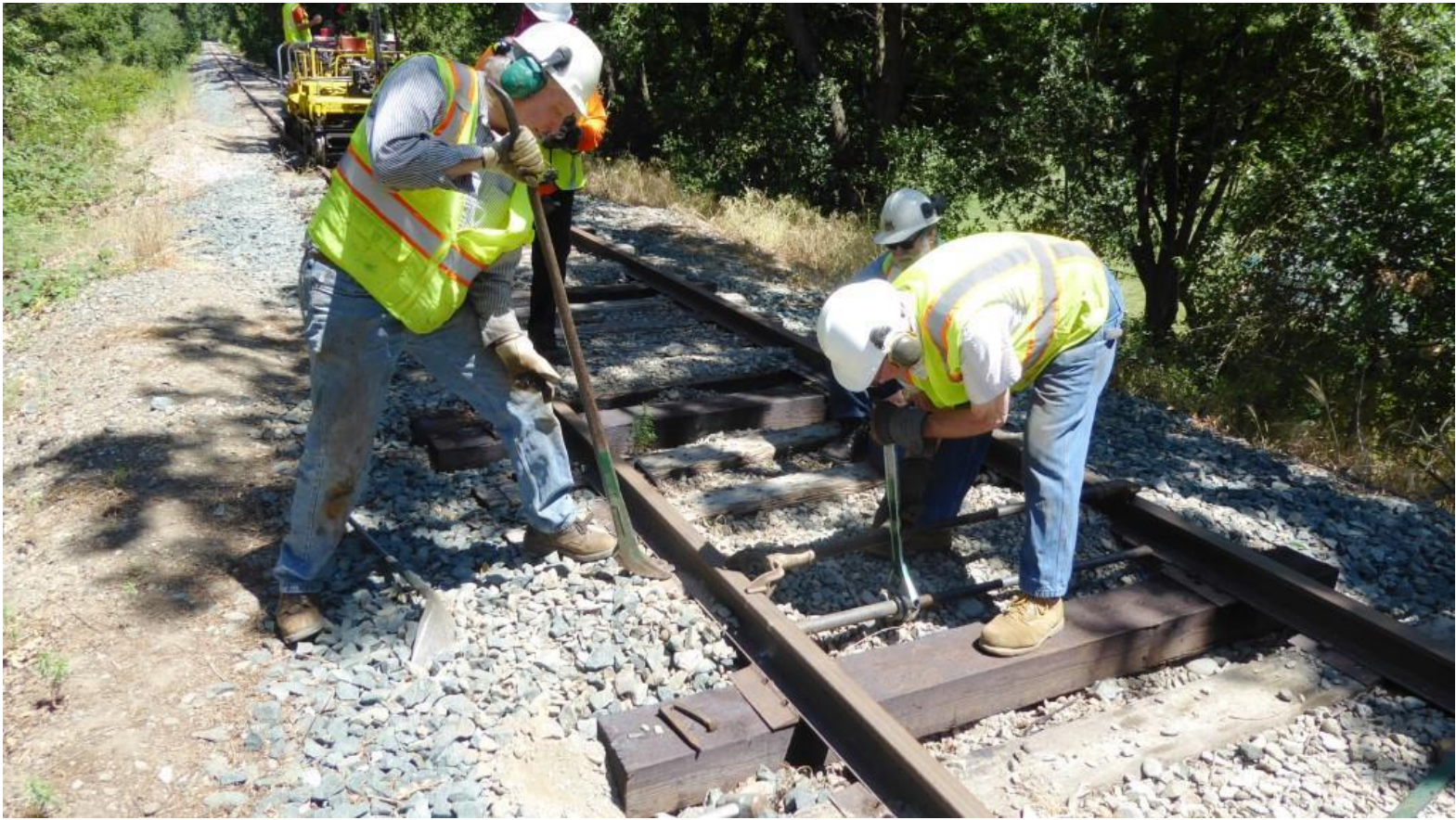
Clem deploys the manual gauger and tightens the nut on its screw-jack with a crescent wrench as Steve pulls spikes on nearby ties
