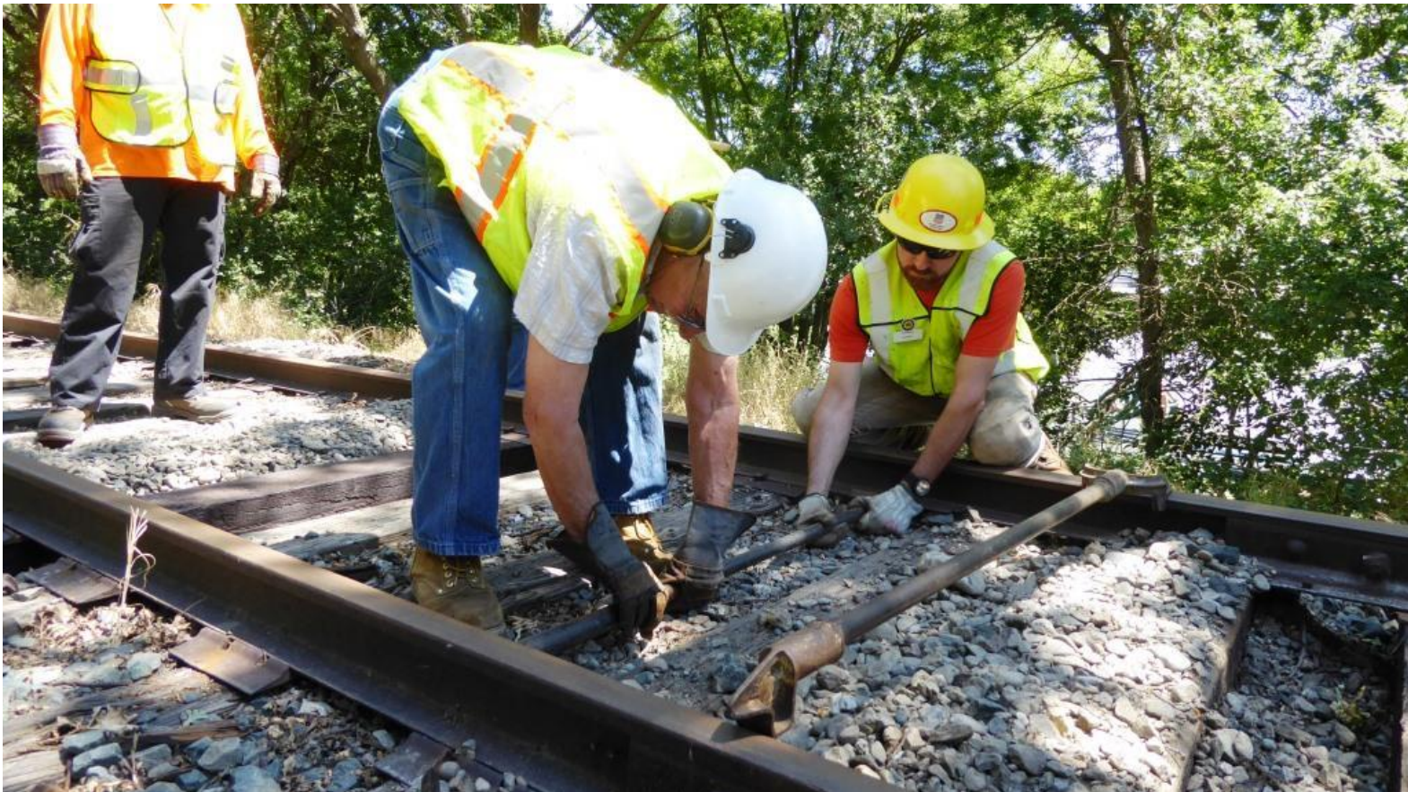
Clem and Chris M. set the manual gauger near the where the pipe-gauge indicates narrow track
