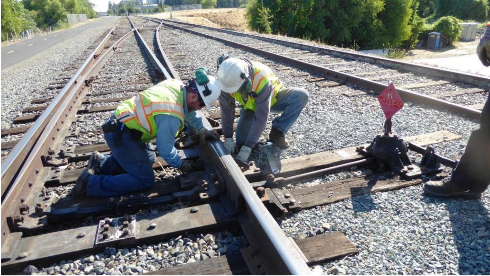
Joe and Steve install a switch-point clamp on the east-point at Switch 13
